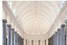
RESTORATION OF ST MEL'S CATHEDRAL
