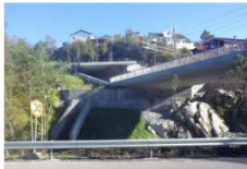
BERGEN LIGHT RAIL - STAGE 3 MOTT MACDONALD IRELAND
