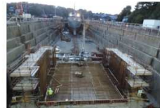
CAPE CLEAR HARBOUR STORM GATES & SLIPWAY
